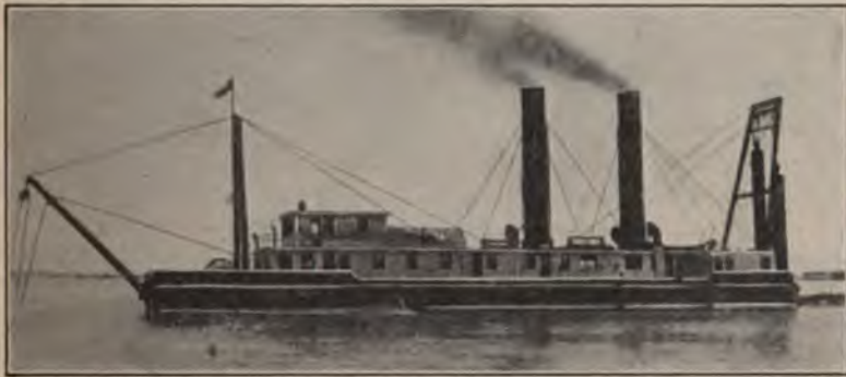
Hydraulic Dredge Operating in Lincoln Park, Chicago.
